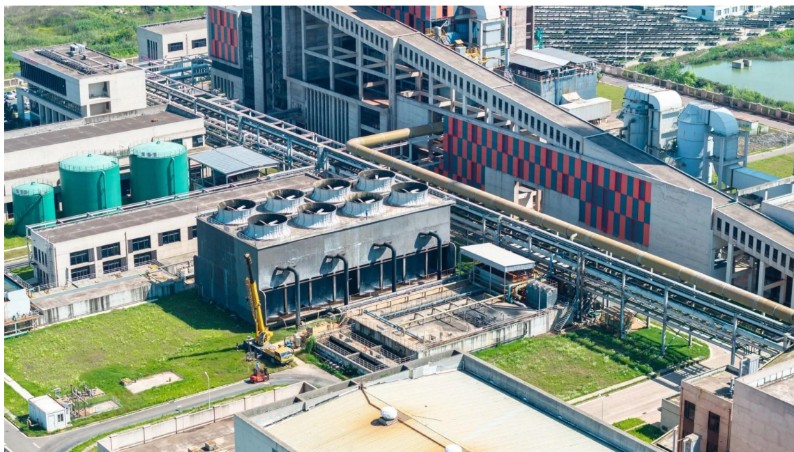
Figure 7. Photograph of a large industrial waste-to-energy facility, illustrating the scale of integrated plant buildings, utility infrastructure and auxiliary systems. Note; facility identity and operating status have not been disclosed.
